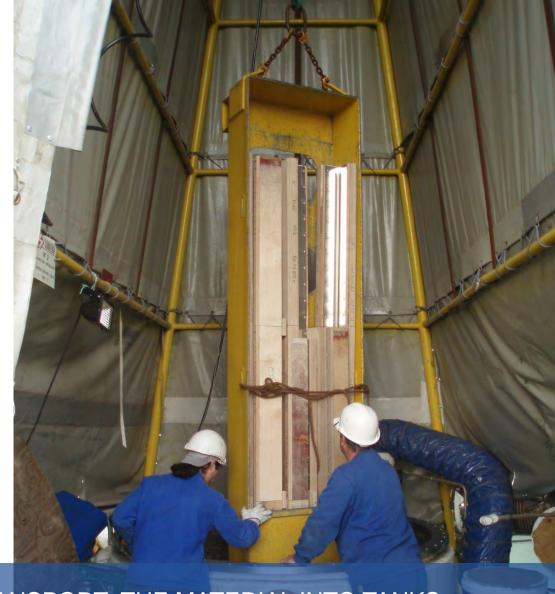
SPECIAL TOOLS FOR TRANSPORT THE MATERIAL INTO TANKS
